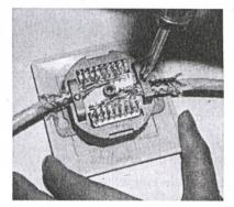
Fasten the screws to secure both the braid and the cable jacket.
